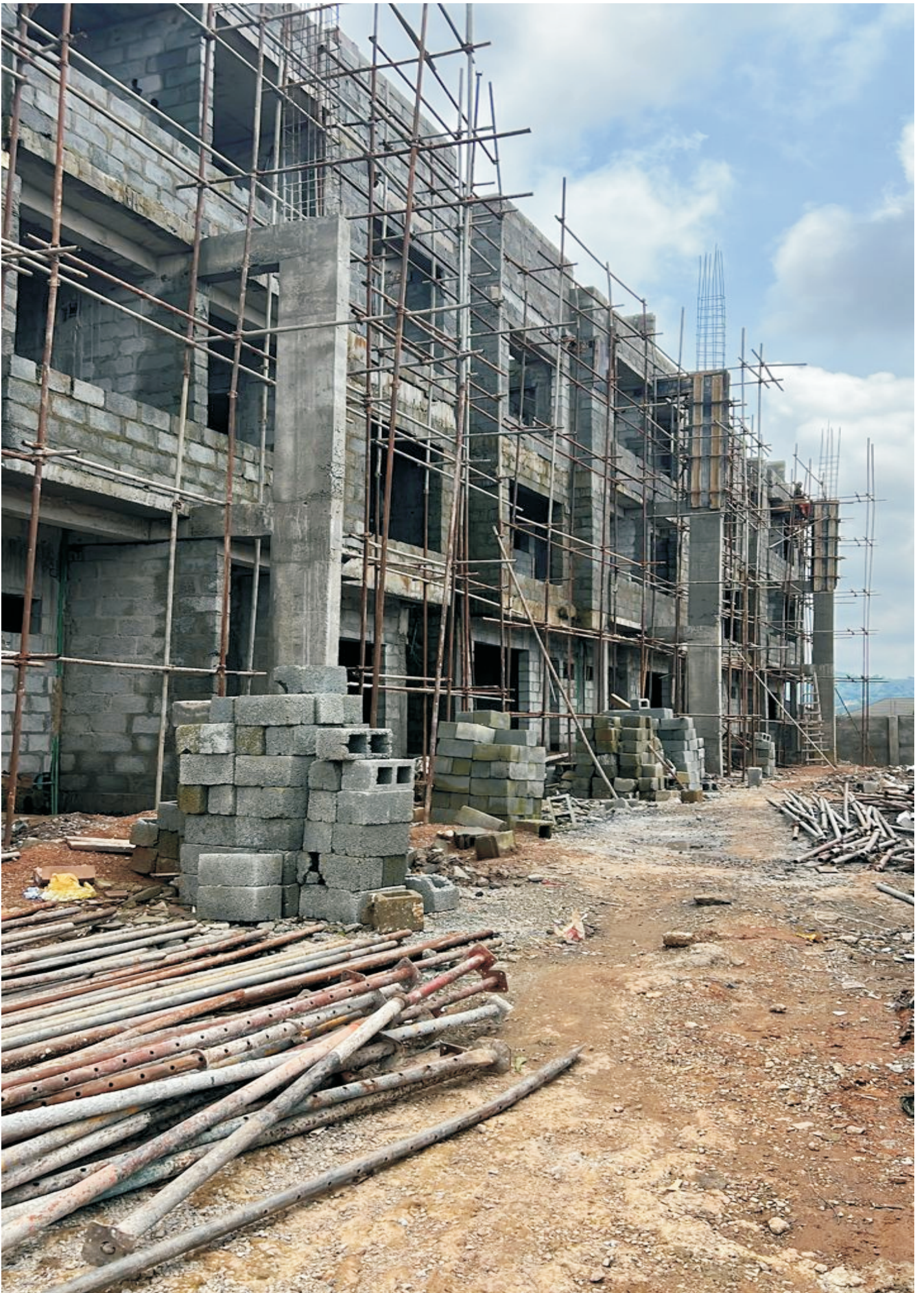
Construction of 6 Unit of Terrace Duplex, Plot 461, Gwarimpa, Abuja.
