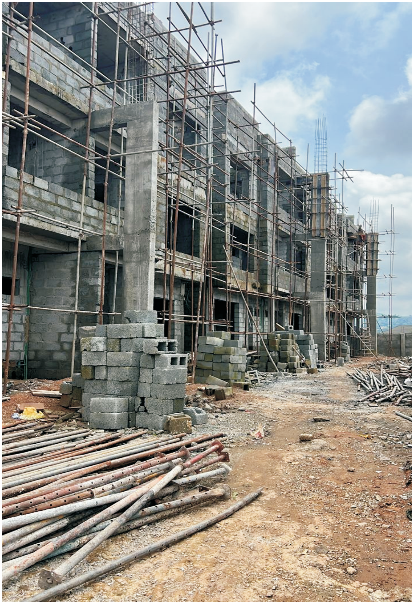
Construction of 6 Unit of Terrace Duplex, Plot 461, Gwarimpa, Abuja.
