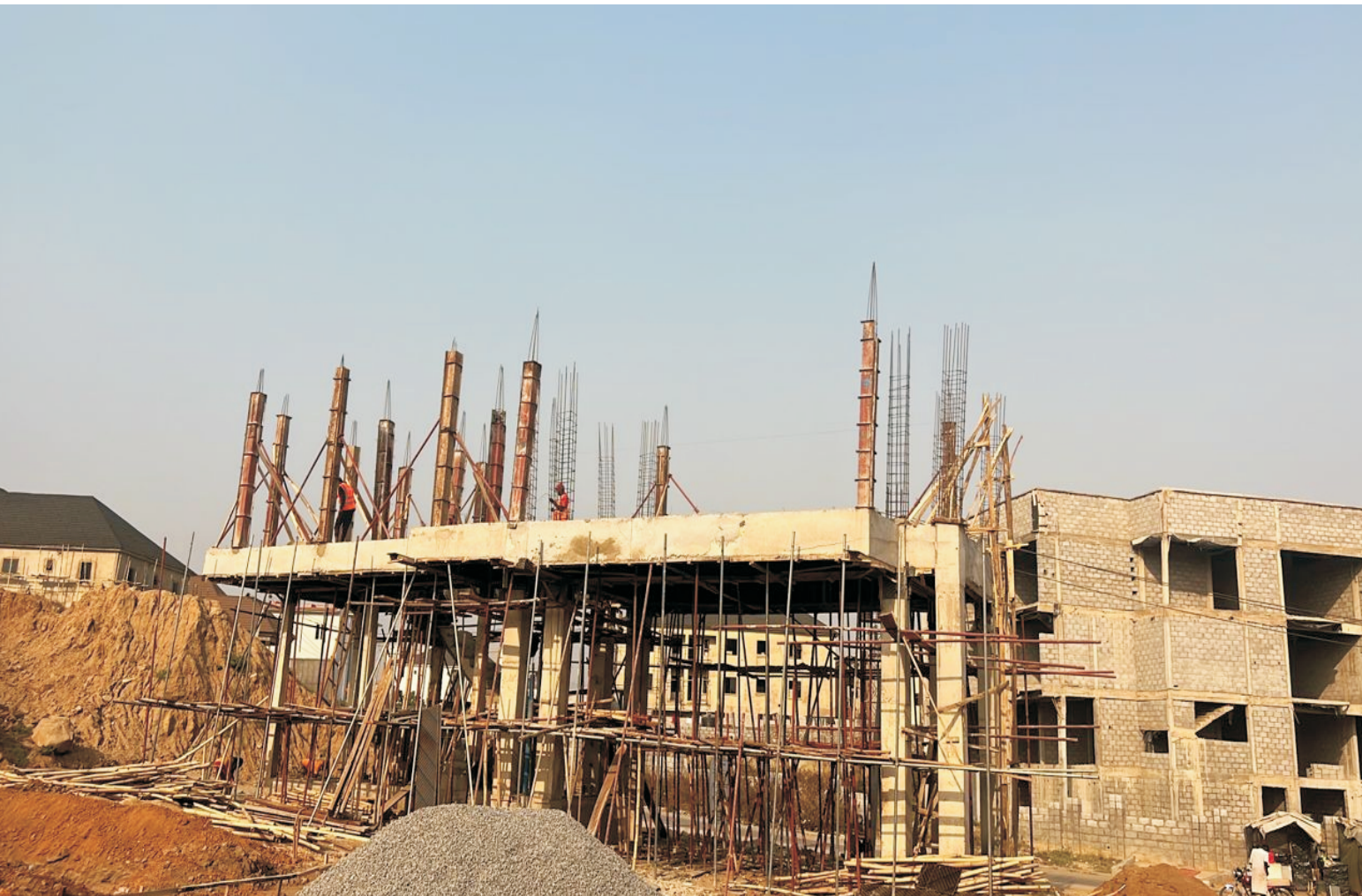
Construction of Gate House, Jahi
