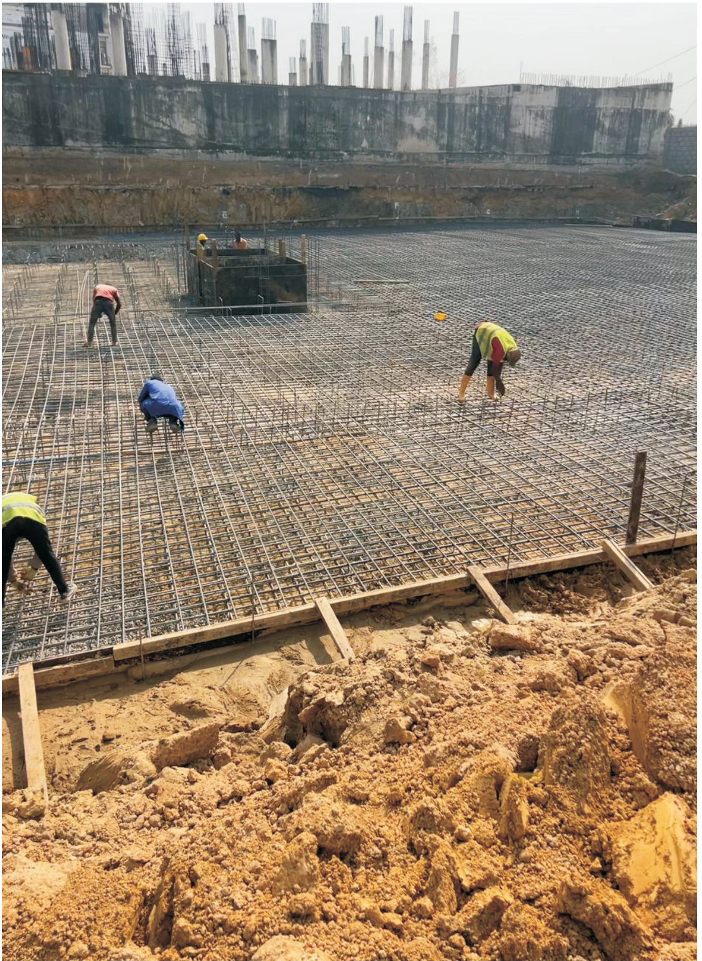
Construction of 60 Unit Shops Plaza, Plot 118 Cadastral Zone, Mabushi, Abuja.
