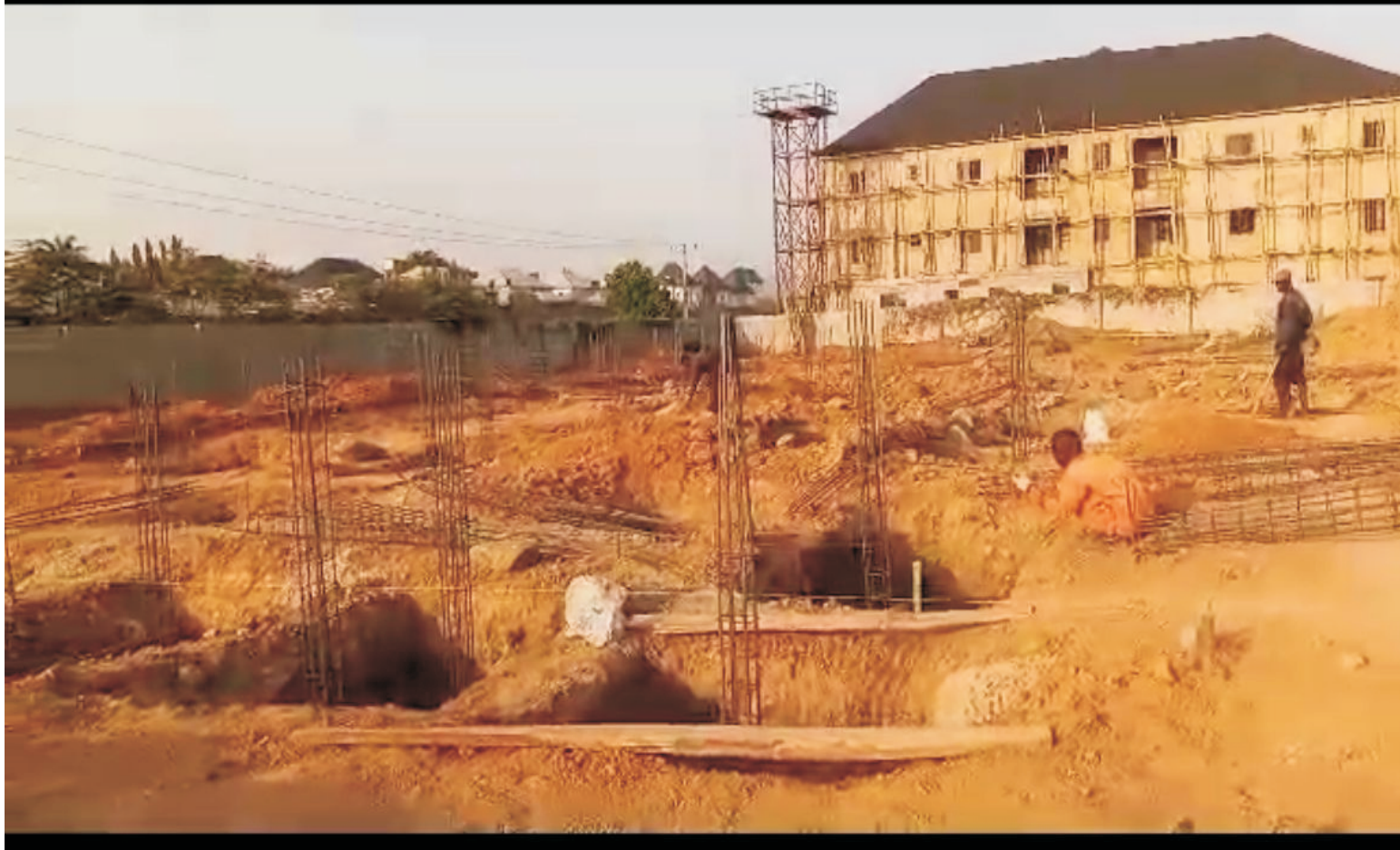
Construction of Gate House, Jahi
