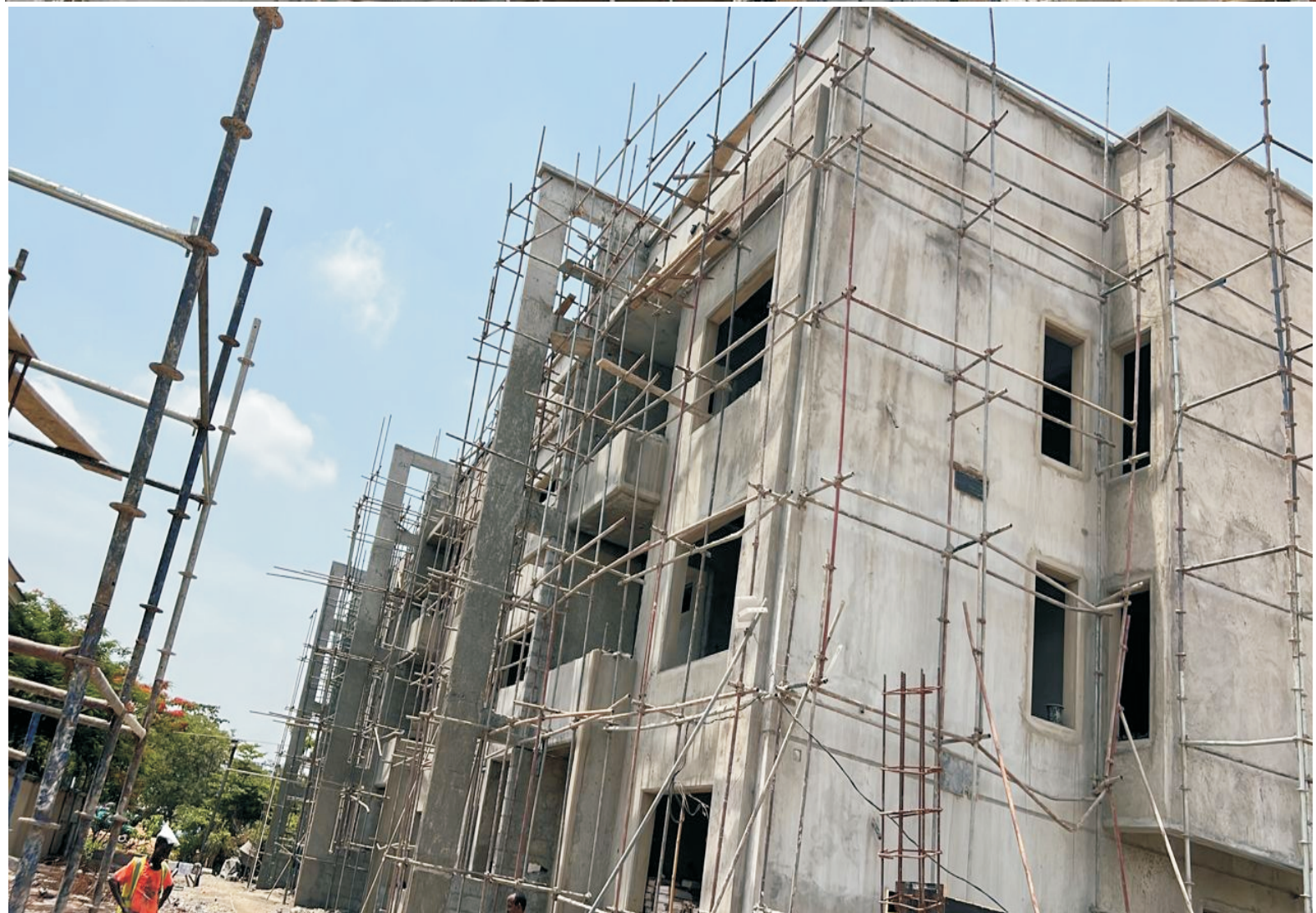
Construction of 6 Unit of Terrace Duplex, Plot 92, Life Camp, Abuja.
