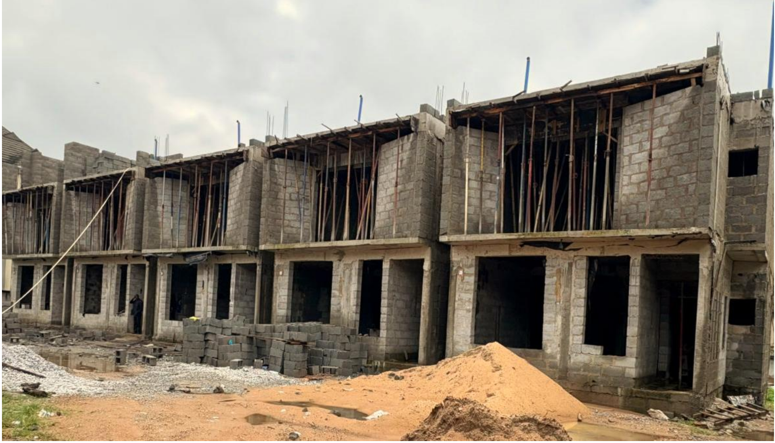
Construction of 5 unit of Terrace Duplex plot 377, Life Camp, Abuja, Nigeria
