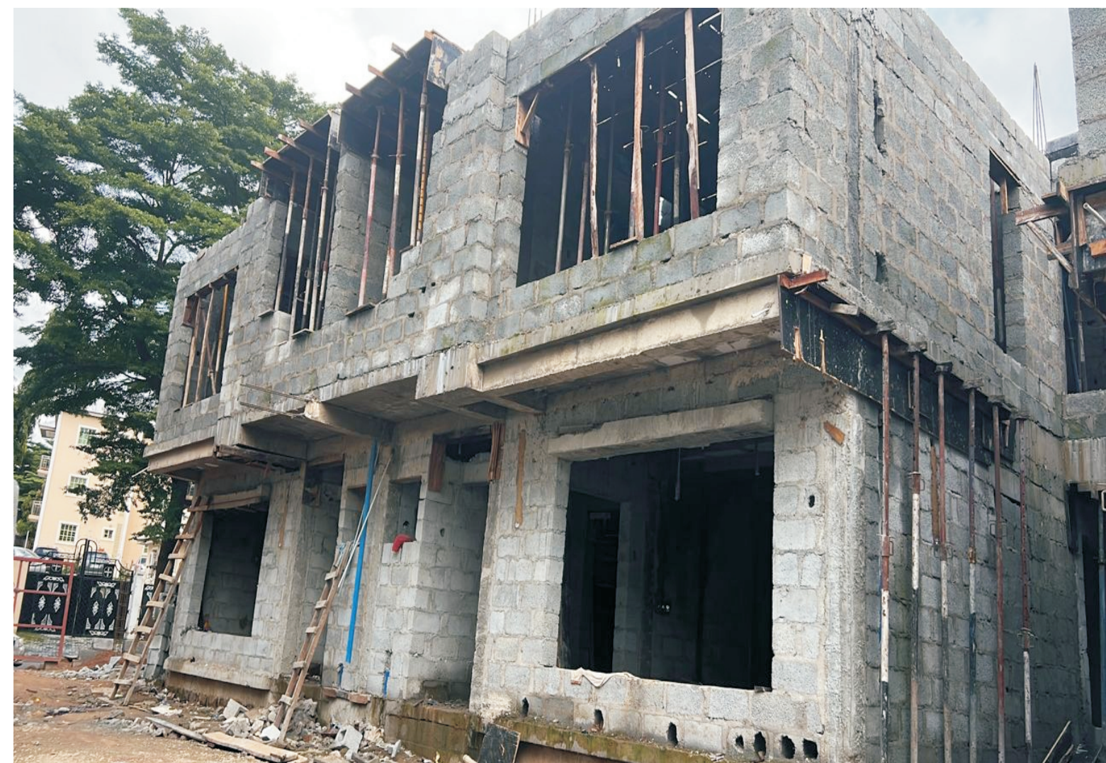
Construction of 4 Unit of Semi-Detached Duplex, Plot 350, Utako, Abuja.
